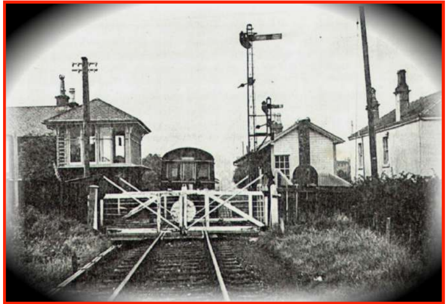
1961: Caledonian box signals at Coalburn. The crossing gates are almost miniatures owing to the narrowness of the road.
